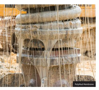
60,000 m³ of soil has been excavated in this project under G3® System polymer slurry with zero quality problem detected in the completed bored pile.
